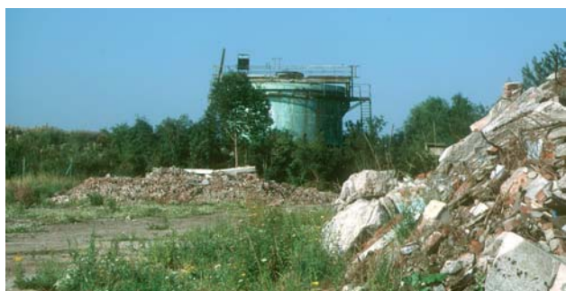
Site pollué Wattrelos Sartel Kullman.
