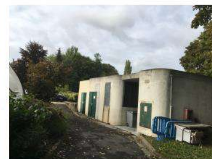
Local technique piscine
