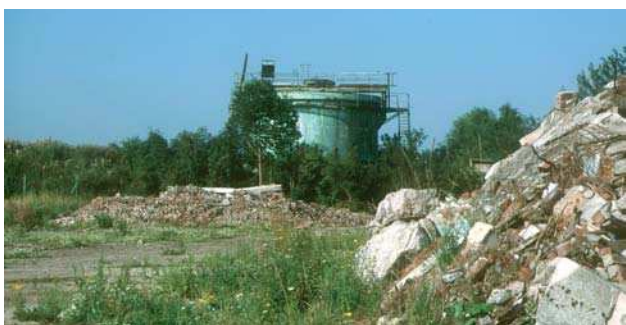
Site pollué Wattrelos Sartel Kullman.
