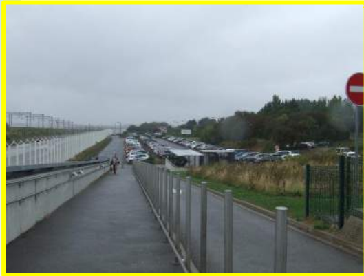
Rampe parking Briqueterie – passerelle
